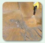
remove / clean any surplus mortar from the surface carefully using more water ...
