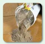
pour the mortar onto the wetted surface in small piles
