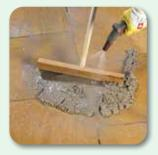
slurry into the joints using a soft water jet and a hard rubber squeegee
