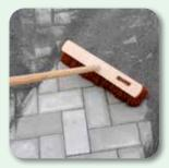
Brush VarioSand into the joints, brush off any surplus material
