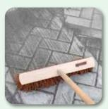
Following, take a second go; put further sand into the joints and compact again. Afterwards brush off residue-free and clear chamfers, if necessary
