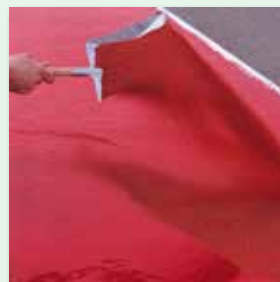
Broadcast aggregate onto the fresh coating
