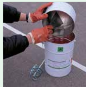
Pour component B into component A and mix thoroughly
