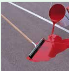
Apply all of the material and spread it with a rubber squeegee
